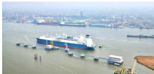
Klaipeda LNG terminal based on FSRU Independence
