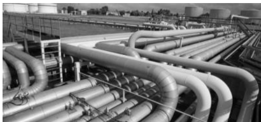
State fuel reserves terminal
